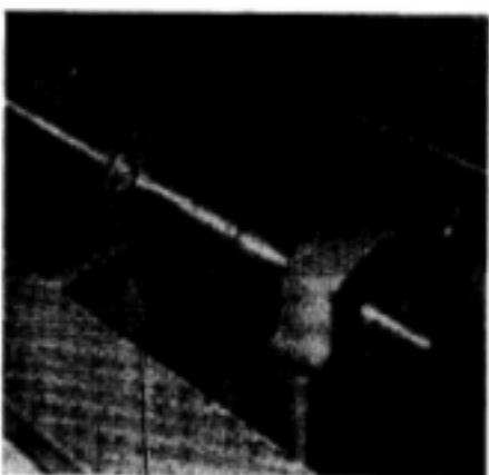
Lubrication oil pipe
